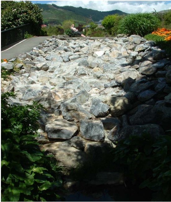
Figure 16: Emergency overflow spillway on Jimmy-Lee Creek at Retention Dam in Washbourne Gardens
