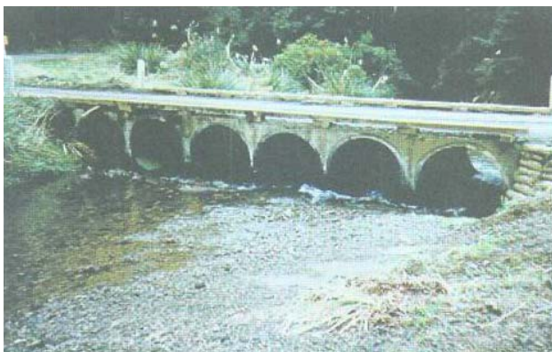
Figure1; A: Top left: A fish-friendly culvert showing the natural stream bed filling the base. Figure B: Top right: The use of spoilers can be used to create resting places for fish that can only sustain short bursts of swimming in high velocity water. Figure C & D: With multiple barrels some can be set deeper to ensure passage at low flows.
