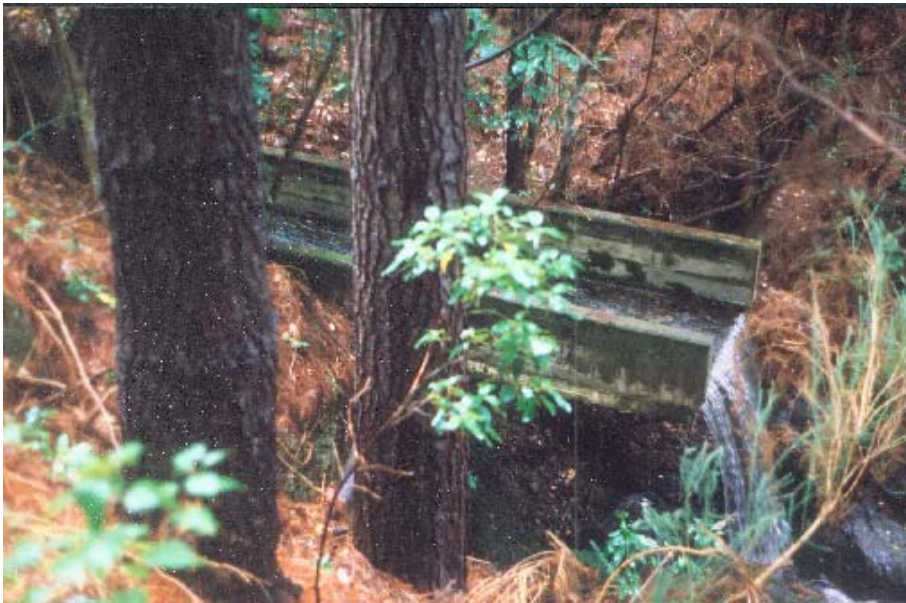
Figure 13: Example of a forestry culvert acting as a barrier to fish passage.
