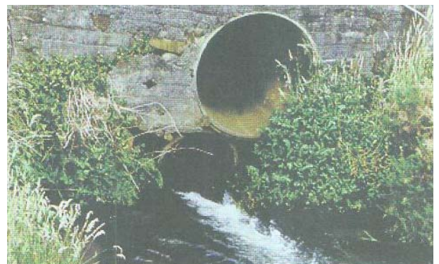
Figure1; A: Top left: A fish-friendly culvert showing the natural stream bed filling the base. Figure B: Top right: The use of spoilers can be used to create resting places for fish that can only sustain short bursts of swimming in high velocity water. Figure C & D: With multiple barrels some can be set deeper to ensure passage at low flows.
