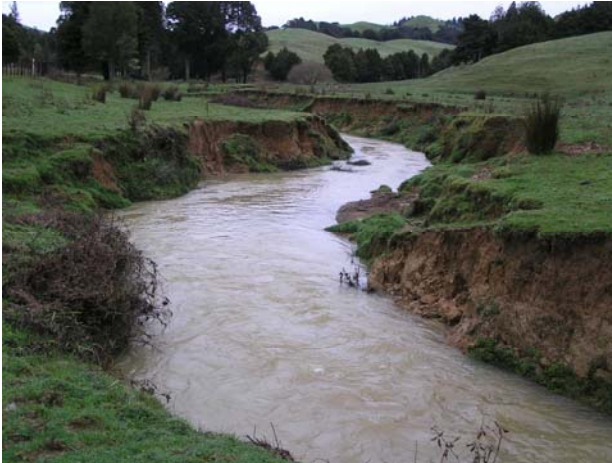
Slab failures, Raglan
