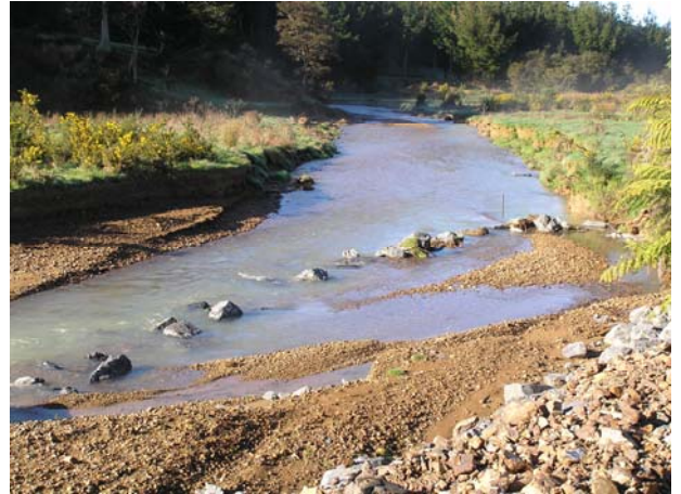
Slab and soil fall failures, Raglan
