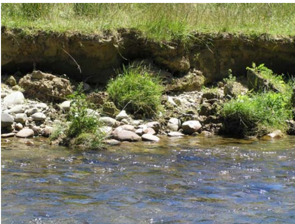
Slab failures, Motueka River
